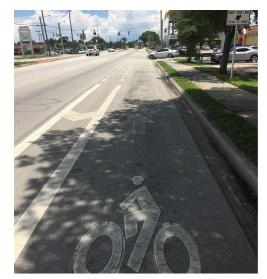
There is a 7' wide bike lane with a 3' foot buffer on SR 80 in Southern Belle Glade. The buffer provides more comfort to bicyclists, however a barrier could provide an added level of safety.
