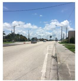
Looking east on SR 80 from US 27, the south curb lane is very wide and has a 10' buffer. The additional lane width and the buffer are adequate to shift the median and provide bike lanes on both sides of the road.
